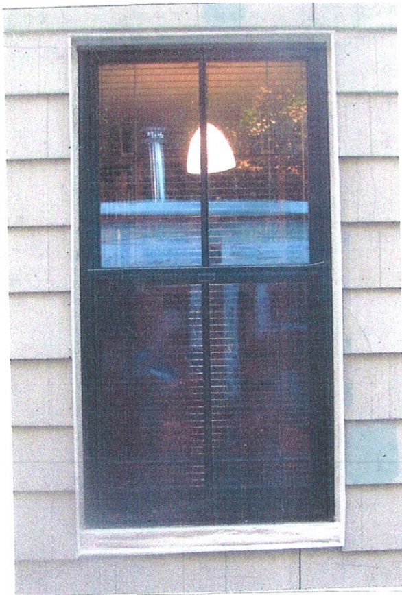
Exterior View of New Pella Window
